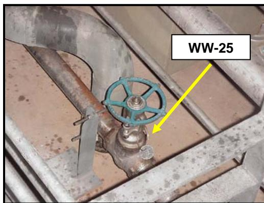
18. Open and Tag 9<sup>th</sup> stage extraction drain (WW-25)
