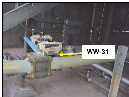
23. Open and Tag CT Inlet Plenum drain valve (WW-31). \_\_\_\_\_
