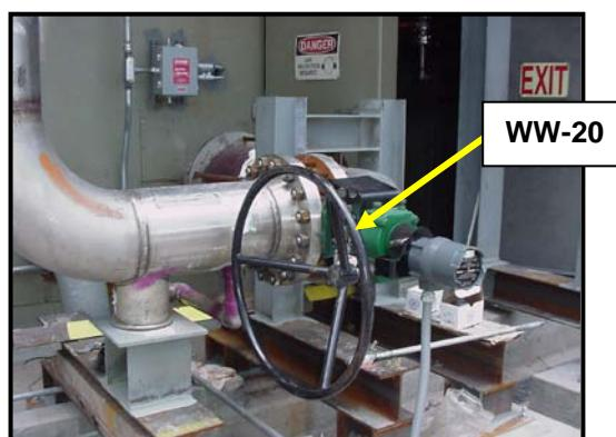
16. Close and Tag Compressor Bleed Heat manual isolation valve (WW-20) \_\_\_\_\_
