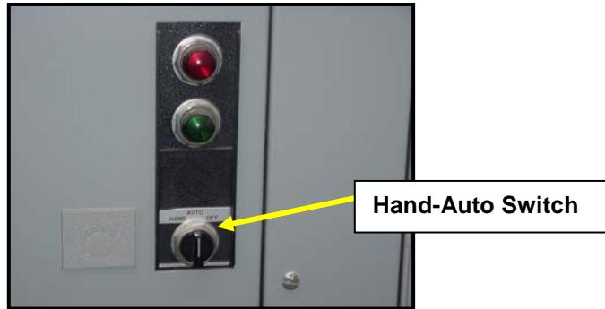
24. With all the low point drains opened and tagged, the last step before releasing the clearance on the LCI is to set both exhaust frame blowers to the HAND position. See photo above.
