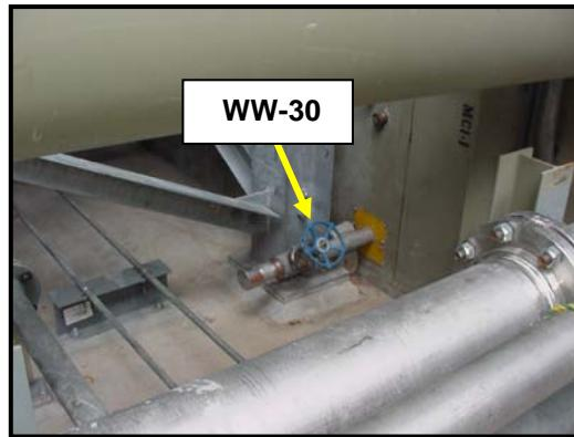
22. Open and Tag 13<sup>th</sup> stage extraction drain valve (WW-30). \_\_\_\_\_
